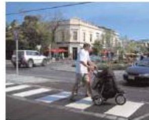
AS THE RADIUS OF THE KERB IS INCREASED, CARS ARE ABLE TO TRAVEL FASTER AND THE OBSTACLES PEDESTRIANS HAVE TO CROSS INCREASE. MAKING WALKING SAFER, HAZARDOUS. KEEP KERB RADIUS TO A MINIMUM AT INTERSECTIONS TO SLOW TRAFFIC AND PROVIDE THE SHORTEST POSSIBLE CROSSING DISTANCES FOR PEDESTRIANS AND OTHER USERS. ENSURE CROSSING POINTS ARE EASILY IDENTIFIED FOR ALL USERS.
