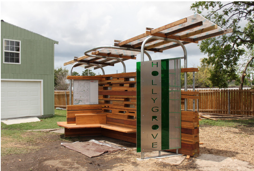
New bus shelter - resident designed and built with recycled material Photo Jason Tudor
